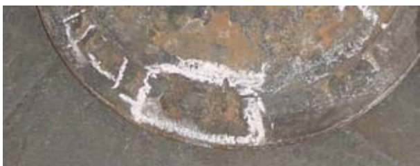
Figure 08: “Cobble stone corrosion” appearance of valve spindle failure through high-temperature corrosion (MC60 Standard-type)
