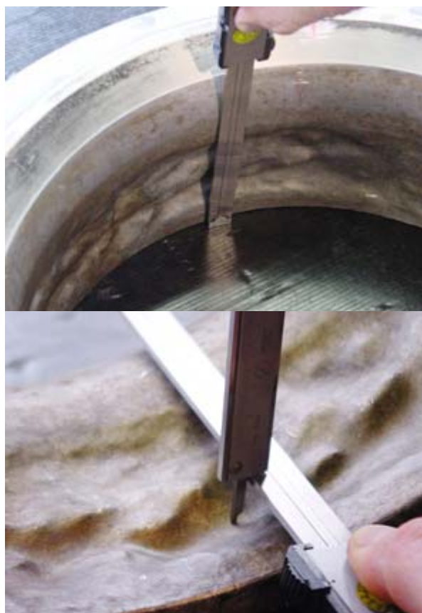
Figure 06: Low temperature corrosion of bottom piece (RTA-type after 28,420 hrs)
