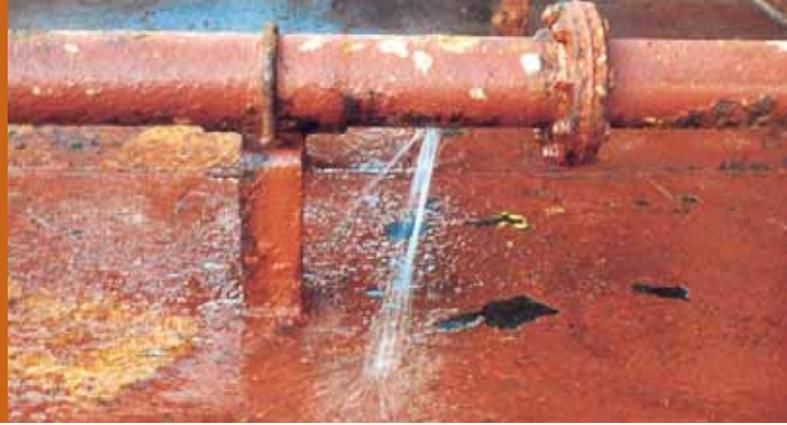
Image: Leaking fire main
