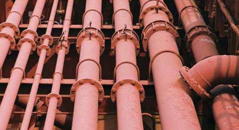
Image: Deck cargo piping on a tanker
