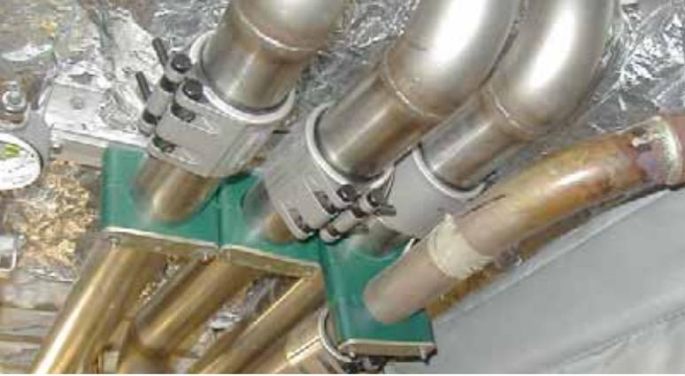
**Image:** Pipes with grip-type joints
